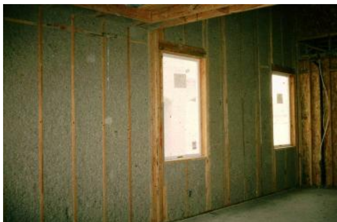
Figure 1.1.9 - Blown cellulose insulation
