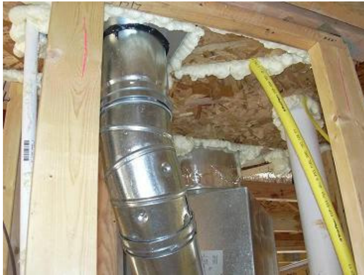
Figure 4.1.4 - Blocking and foam air sealing in chase
