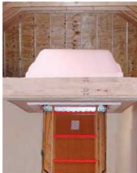
Figure 5.2.4 – Insulated box made specifically for attic drop-down stair
