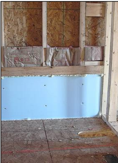
Figure 2.1.3 – Architectural detail of tub installation with complete air and thermal barriers
