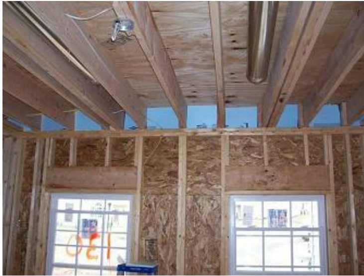
Figure 2.6.3 - Appropriate blocking at intersection of flat porch roof and conditioned space
