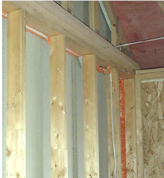
Figure 6.1.4 - Example of properly air sealed common wall with fire-rated caulk (in red)
