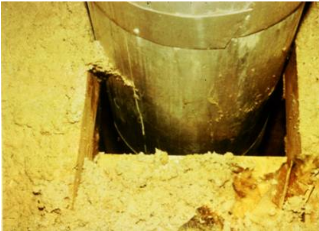
Figure 4.1.1 – Duct penetration to attic that needs blocking
