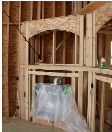
Figure 2.2.1 - Fireplace installed without air barrier
