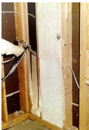
Figure 1.1.10 - Spray foam insulation
