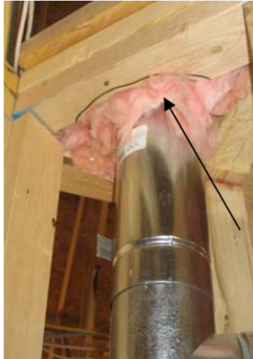
Figure 4.3.1 - Insulation improperly used as an air barrier
