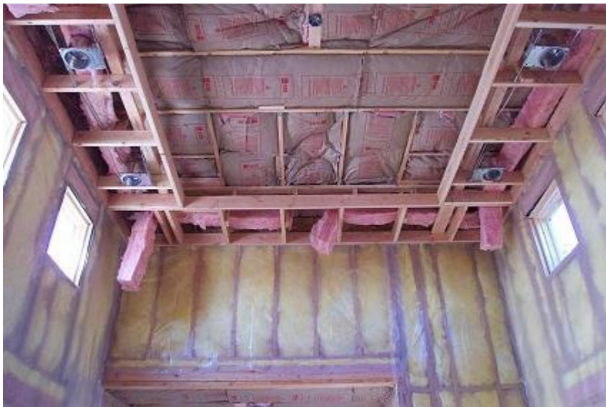
Figure 5.3.1 - Improperly installed insulation over a dropped ceiling
