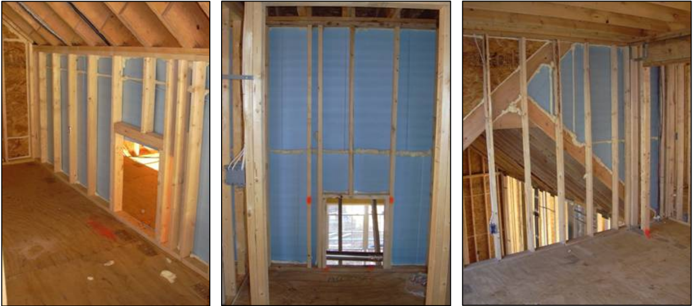
Figure 2.4.3 - Examples of properly blocked and air sealed attic knee walls
