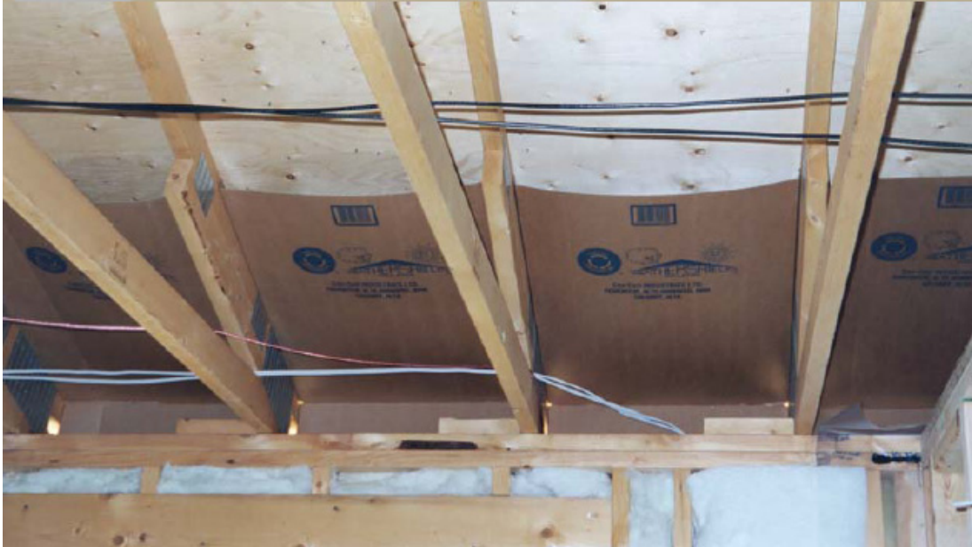
Figure 1.3.2 - Cardboard baffles
