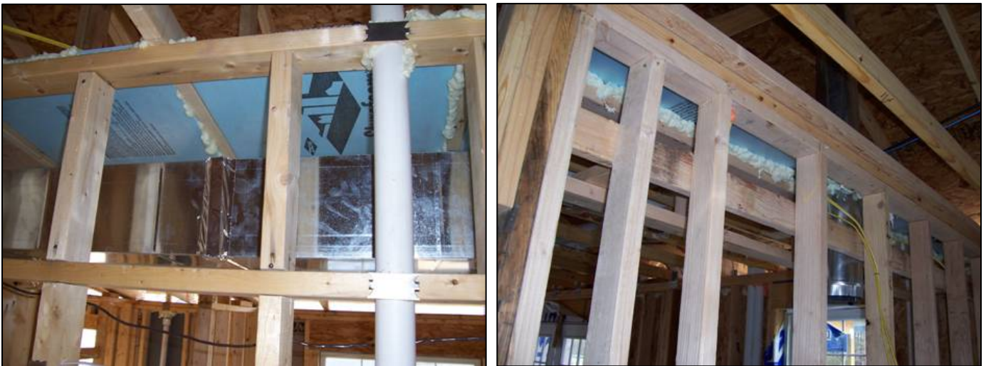
Figure 5.3.4 - Air sealed soffits
