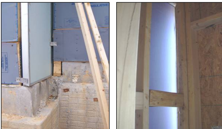
Figure 6.1.2 - Poorly sealed common wall
