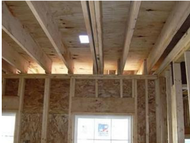
Figure 2.6.1 – Air barrier missing at porch roof
