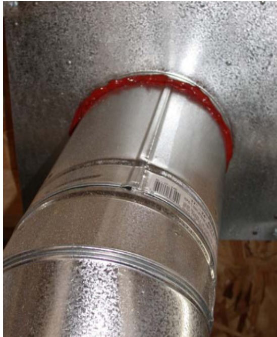
Figure 4.3.3 - Fire-rated caulk around a flue shaft
