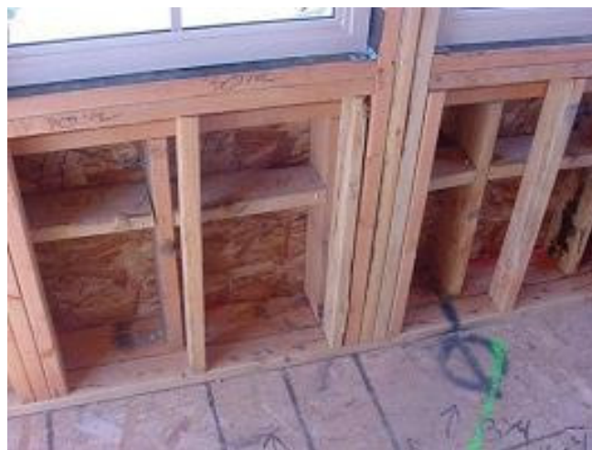
Figure 2.8.3 – Example of a double wall
