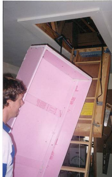
Figure 5.2.3 - Option for insulation of drop-down stair
