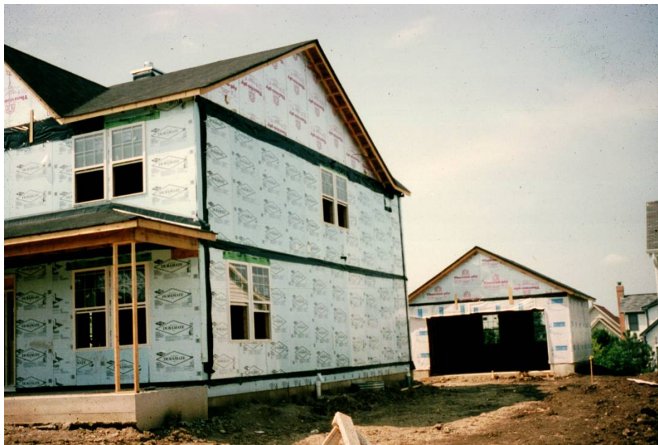
Figure 1.6.3 – Complete thermal break with rigid insulation sheathing
