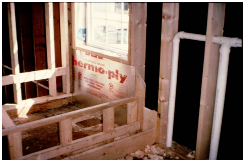
Figure 2.1.3 – Architectural detail of tub installation with complete air and thermal barriers
