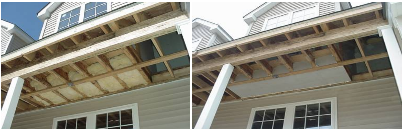
Figure 3.2.5 - Proper installation of insulation under a cantilevered floor
