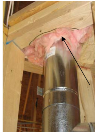
Figure 4.1.2 – Duct shaft with ineffective air barrier (insulation)
