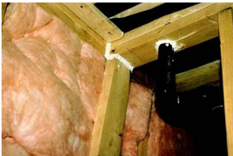
Figure 4.2.2 - Caulking around piping penetration
