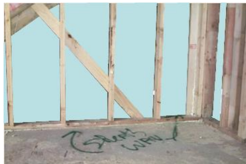
Figure 2.4.5 – Attic knee wall with exterior air barrier
