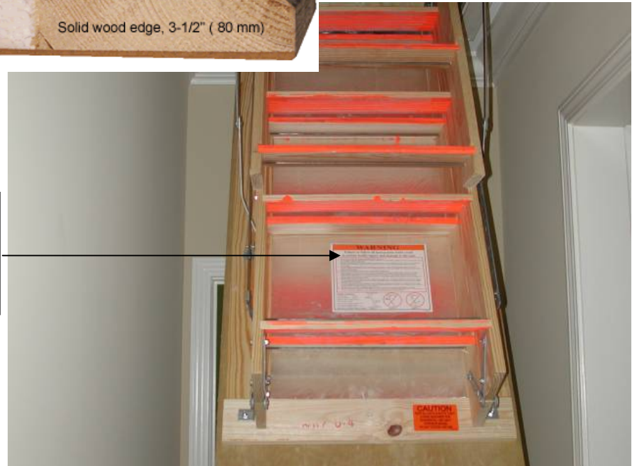
Figure 5.2.3 – Pre-insulated/sealed attic drop-down stair assembly
