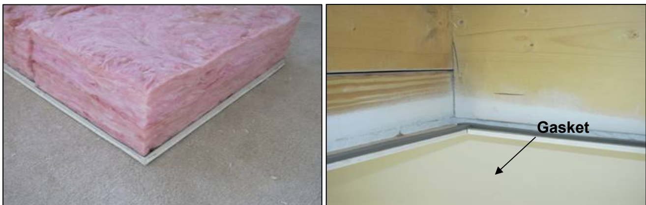
Figure 5.1.2 - Example of properly insulated and sealed attic hatch
