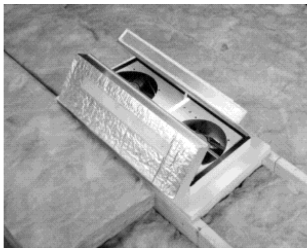
Figure 5.5.2 - Whole-house fan with built-in cover
